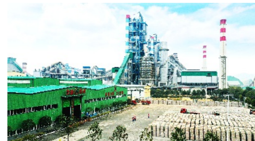
武穴工业园内，由水泥窑烟气 CO2 吸碳制砖自动化生产线生产的环保砖 In Wuxue Industrial Park, concrete bricks produced by production line using CO2 discharged from cement kiln
